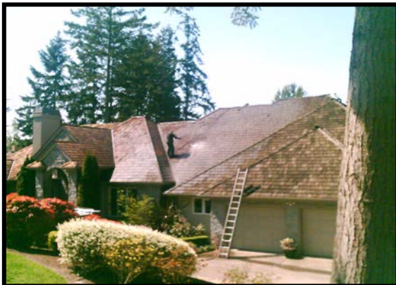
Pressure Wash to Remove Old Moss and Dirt
