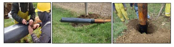
Slip the barrier wrap on to the pole. Snug it up using the double-sided tape that is affixed along the edge. It is preferable to set the pole then trim the barrier wrap to a height of 6" above groundline. After final set depth has been determined, wrap the self-fusing silicone tape around the pole and barrier to tightly seal the top. Applying the final top seal before setting the pole is acceptable but exact knowledge of final set depth is critical to assure proper installation.
