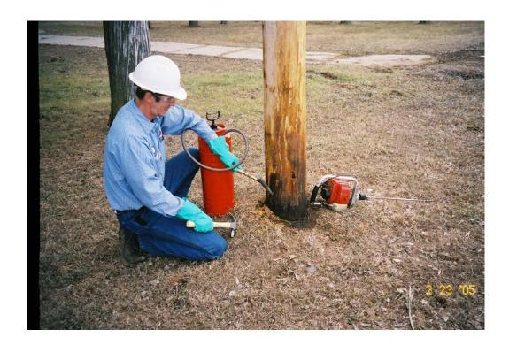
Copper Naphthenate solution is injected under pressure into poles that have decay or insect voids present. After identifying the void area, preservative is applied using a special nozzle. The oil-based preservative penetrates deeply into all areas and will protect against future biological attack. A contact insecticide may also be added.
